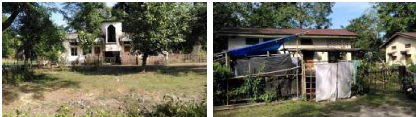
Figure- Site photographs of the existing structures
