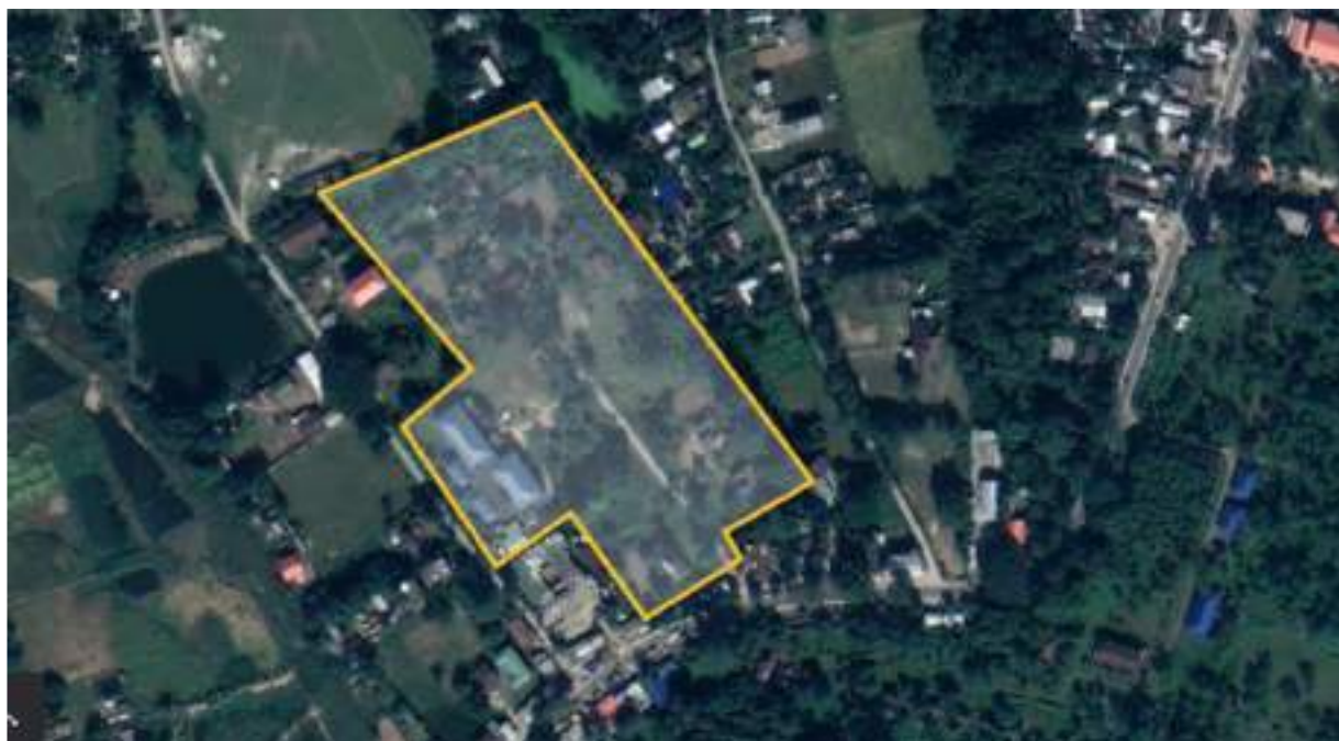
Figure 2.1: Google image of the project site
