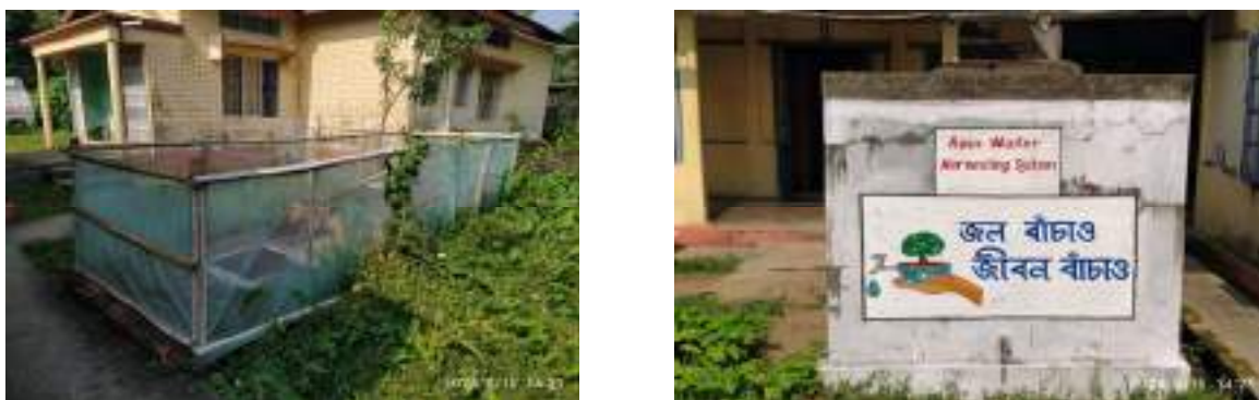
Figure 2.2: Existing site photographs of the project site
