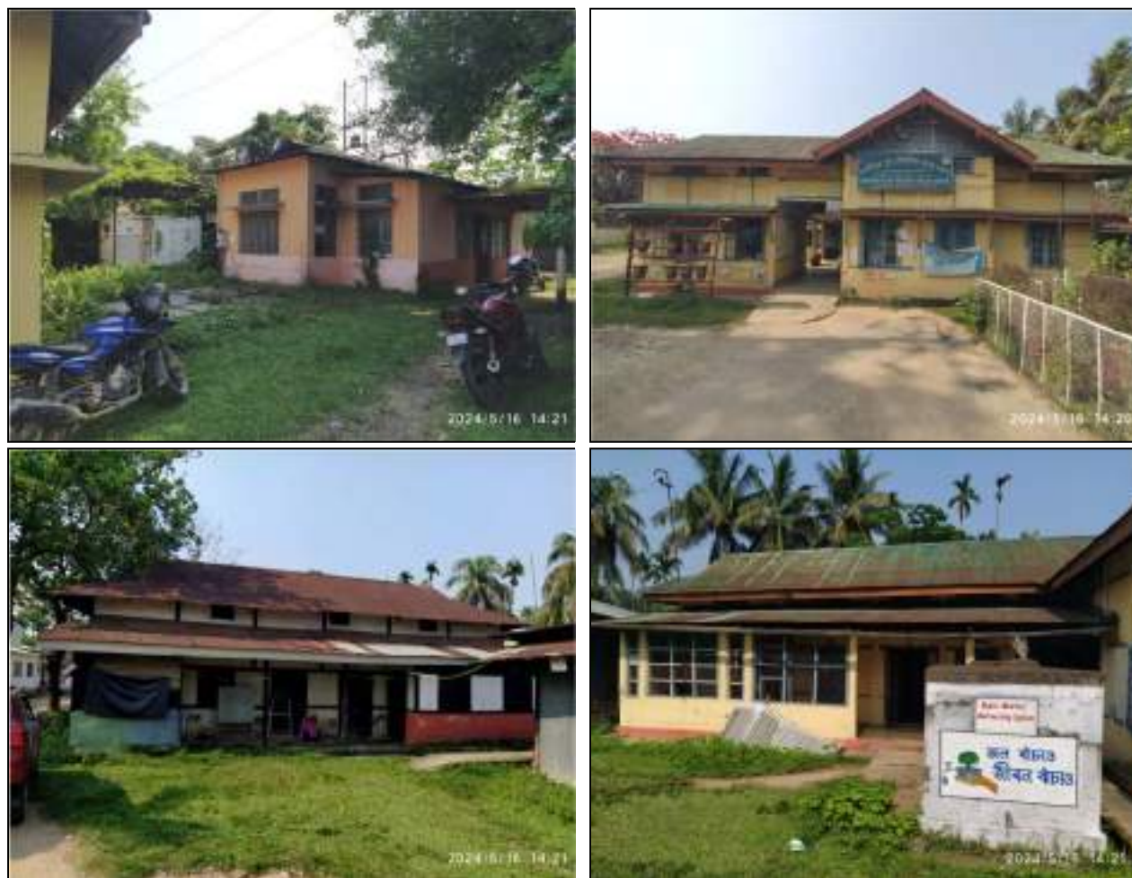
Figure 1- Site photographs of the existing structures
