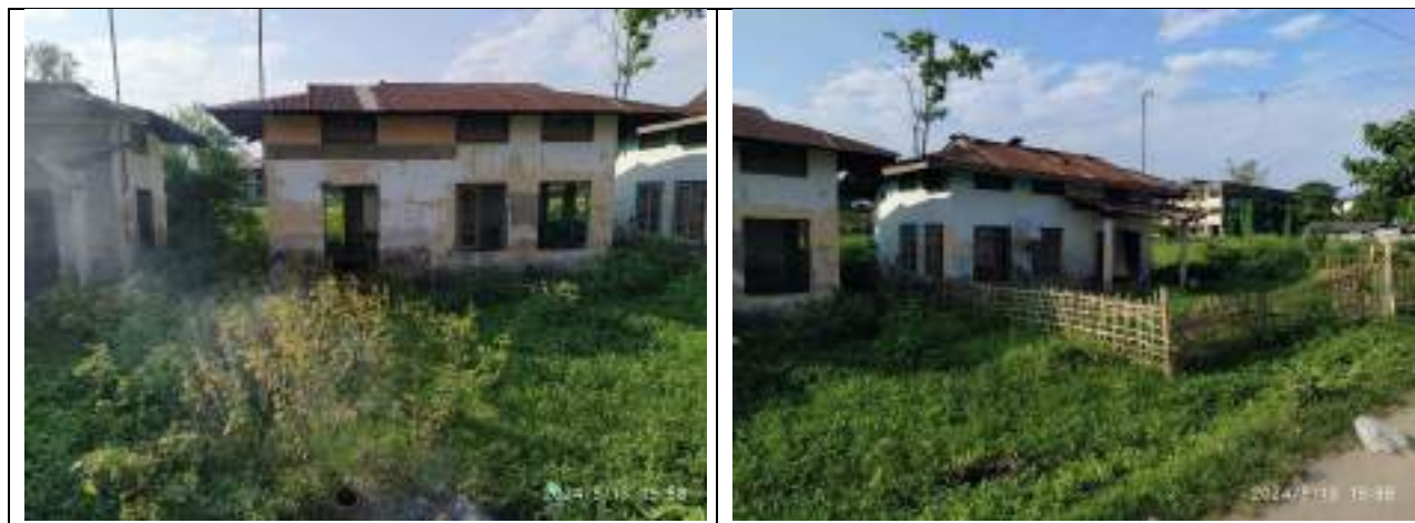
Figure 1. Site photographs of the existing structures
