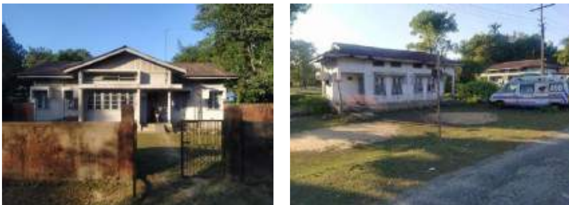
Figure1. Site photographs of the existing structures
