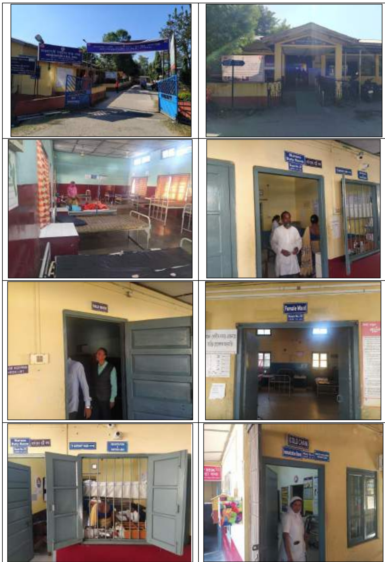
Figure 2.2: Existing site photographs of the project site
