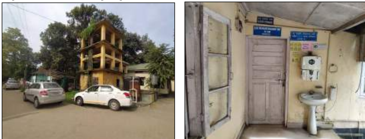
Figure 4.8: Source of Water at Project site
