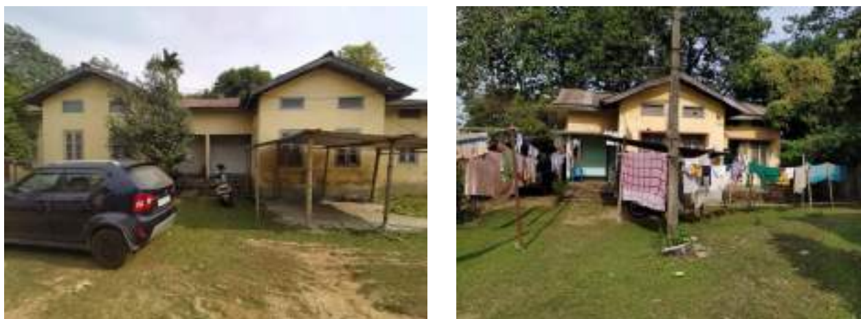
Figure- Site photographs of the existing structures
