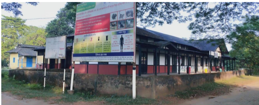
Photograph-2: Existing British Era Hospital Building
