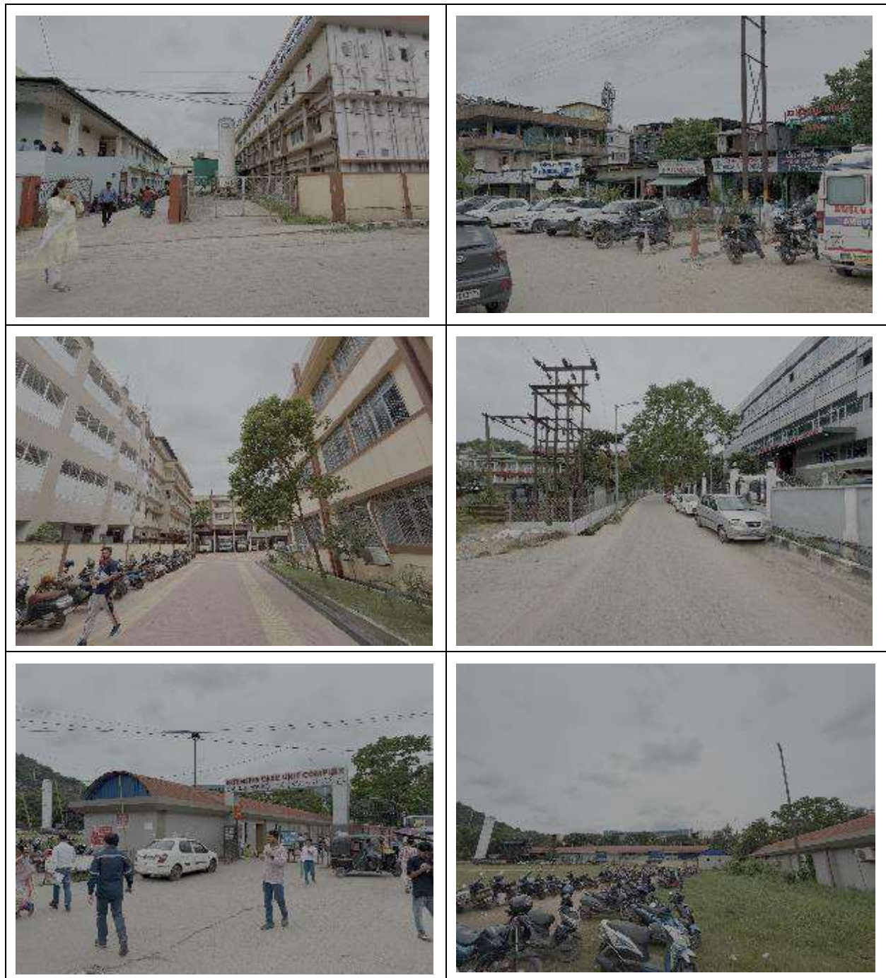
Figure 2: Existing Condition of the Proposed Site for GMCH Redevelopment
